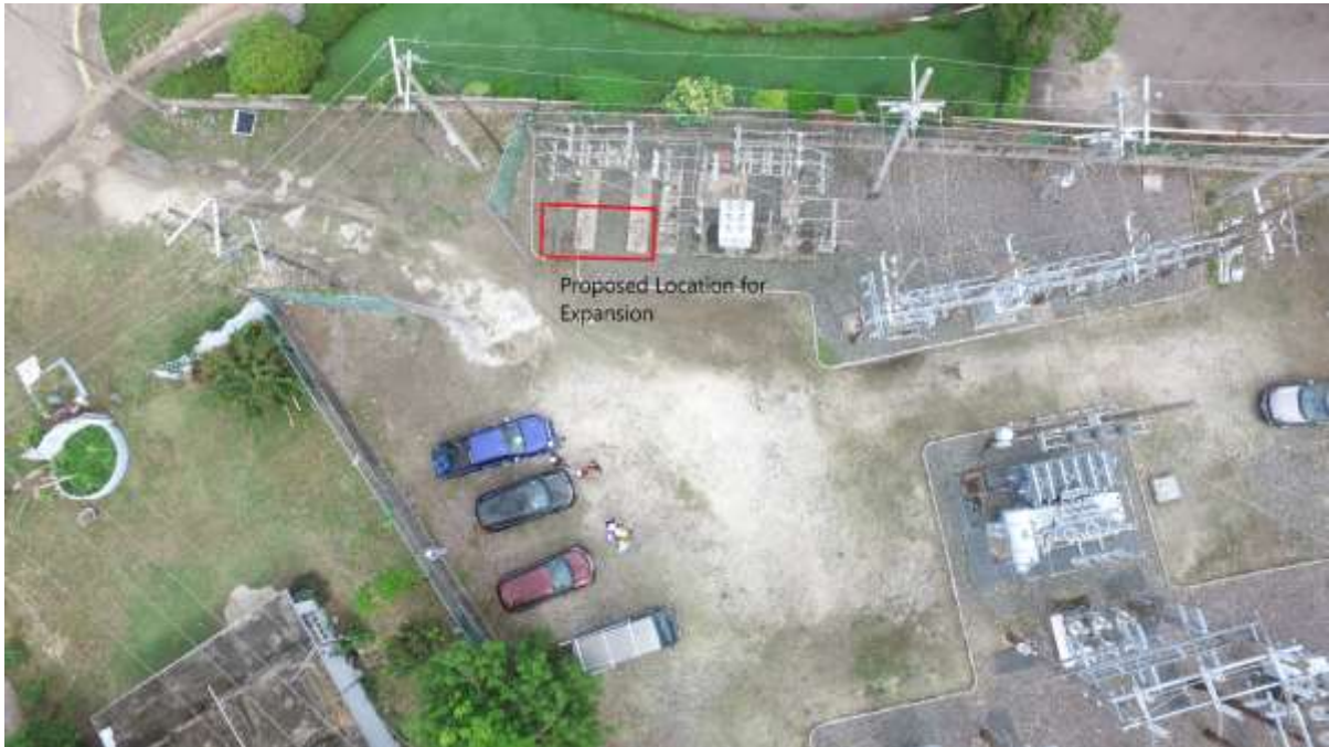
Figure 3: Cardiff Hall Substation Aerial View
