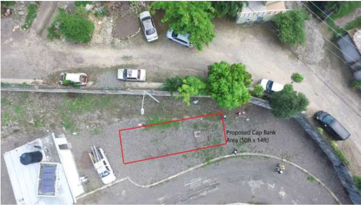
Figure 1: Ocho Rios Substation
