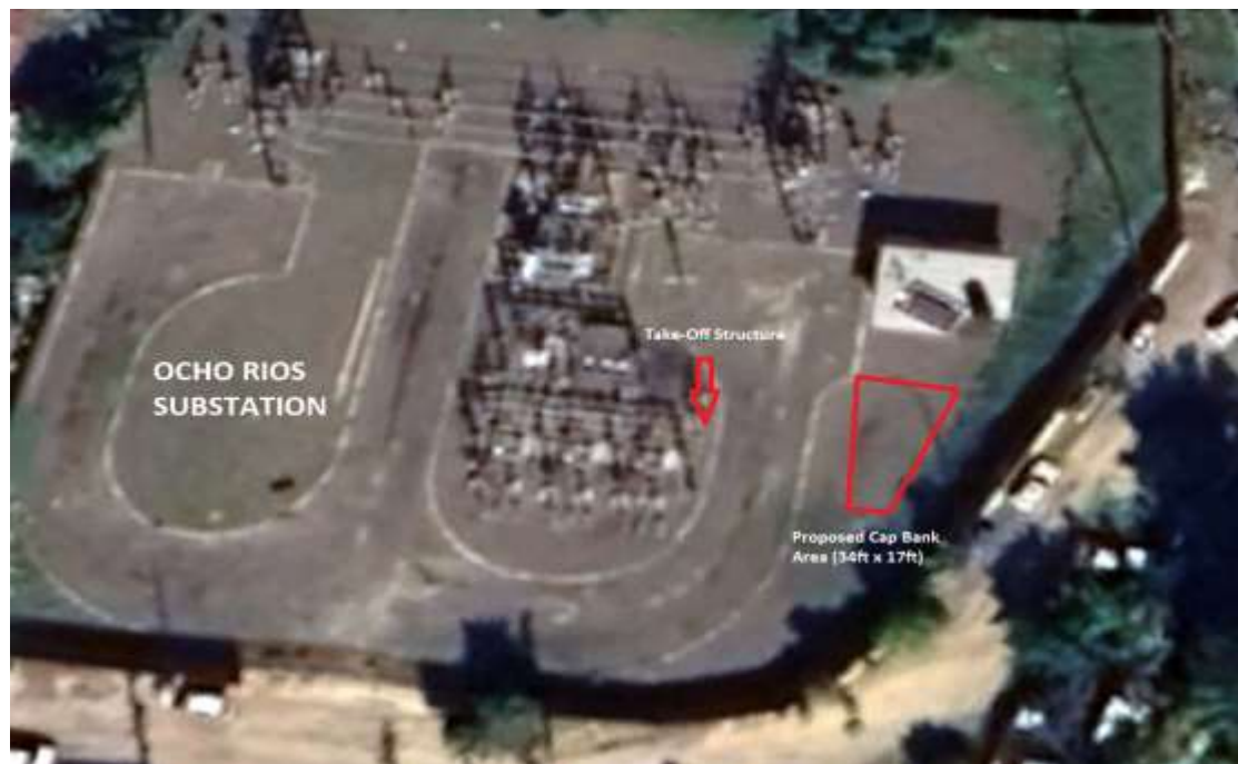
Figure 1: Ocho Rios Substation
