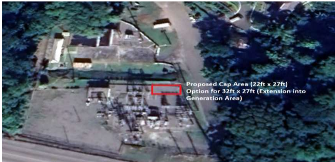
Figure 2: Roaring River Substation
